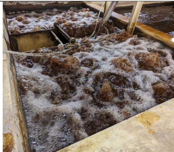
Figure 4 – Bead chamber air scour after a few hours of increase permanganate additions.
